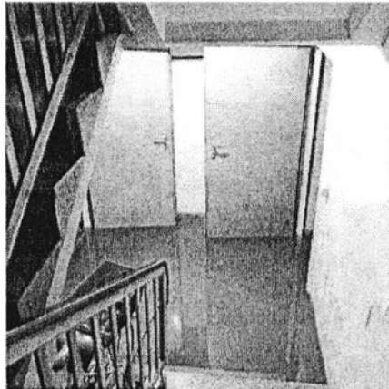
Toronto received more than 4,700 basement flood complaints during and after the July storm, totaling over $850 million in insurance claims across the GTA.
