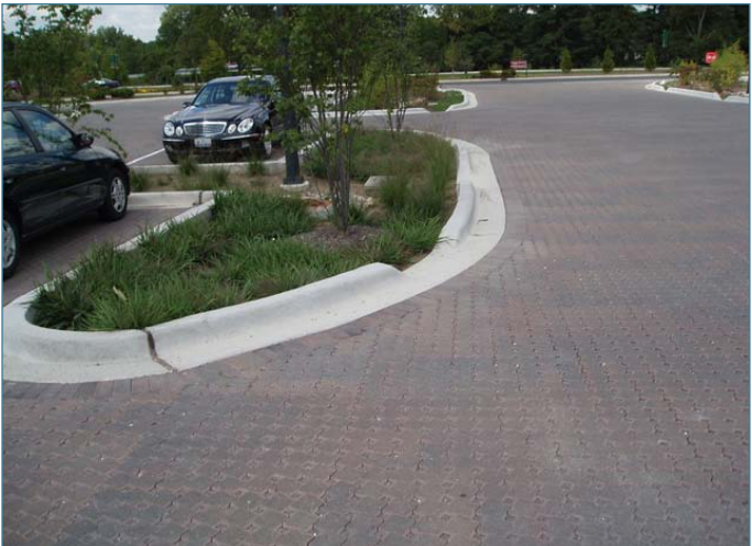
Permeable pavement and stormwater retention/infiltration islands
