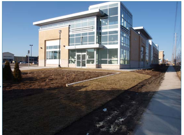
A large format retail establishment with commercial, street-related buildings at the street-edge
