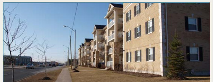
Street-related residential apartment building
