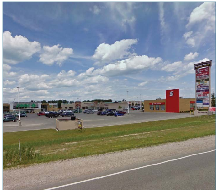
St. Clair Shores is a major commercial/retail anchor within the Lakeshore West Mixed Use Node
